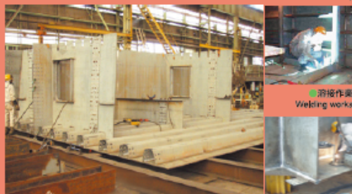
●組立作業 Assembly works
