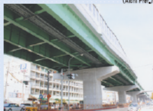
●八州工区 / 名古屋高速道路公社(愛知県) Yaguma Area Highway Bridge Nagoya Expressway Public Corporation (Aichi Pref.)
