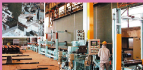
●I 桁組立 I Beam Assembly
