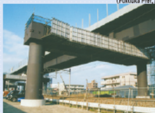
●久米松原Bi橋脚 / 国土建設・運輸施設整備支援機構(福岡県) Kurume-Matsubara Bi Pier / Japan Railway Construction, Transport and Technology Agency (Fukuoka Pref.)
