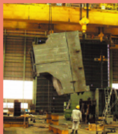
●箱桁反転 Box Girder Reversing
