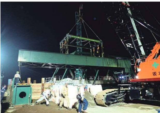
写真-20 A1工事桁撤去
